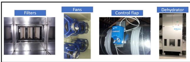
Figure 2. Pictures of different HVAC elements
